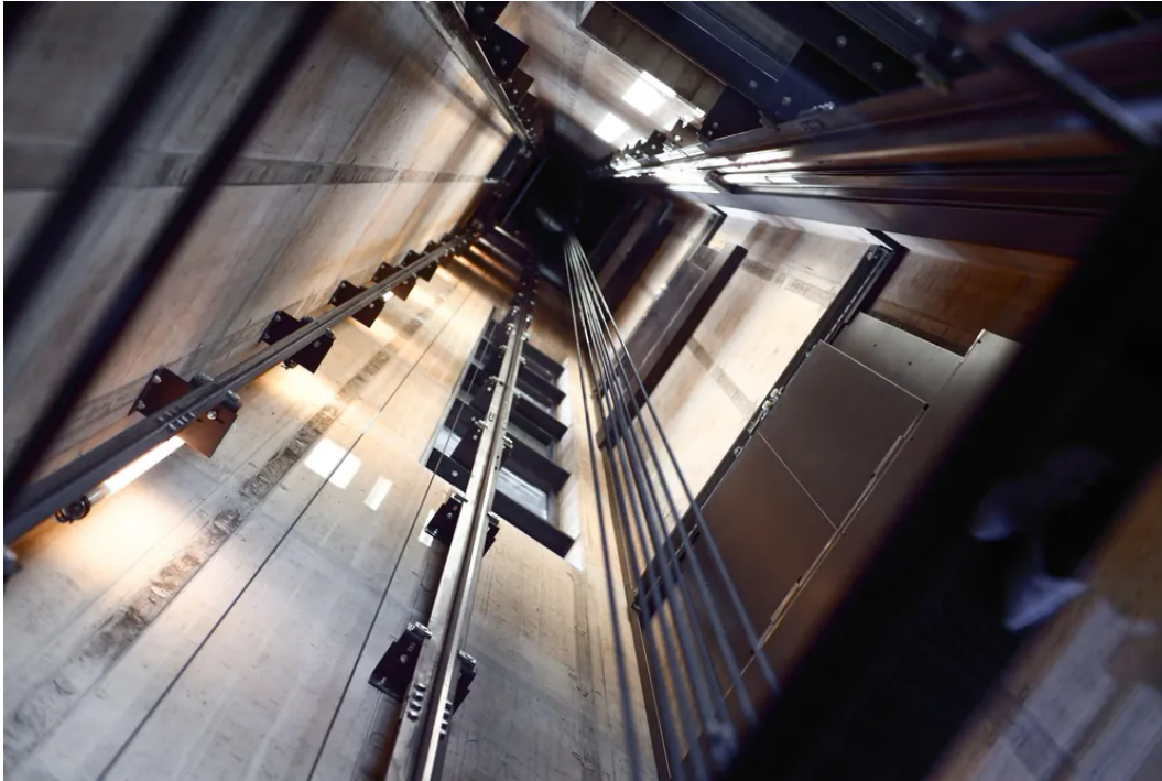
Elevator shaft interior showing rails and cables used for regenerative braking energy recovery
