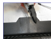
Cut holes to allow cable access
